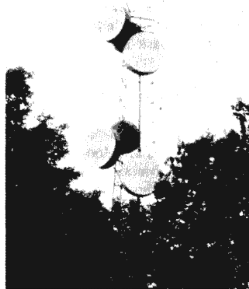
Figure 1.2 A microwave relay tower on which are mounted several radome-enclosed paraboloidal reflector antennas.
